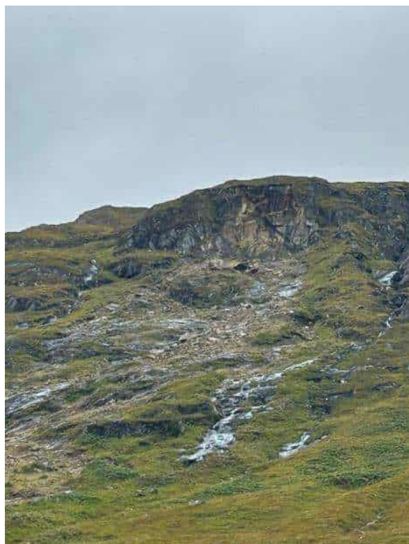
Photo 1: Area of rockfall at Leac Doire Lochaidh. Taken from NGR NH 06933 02893, facing north.
