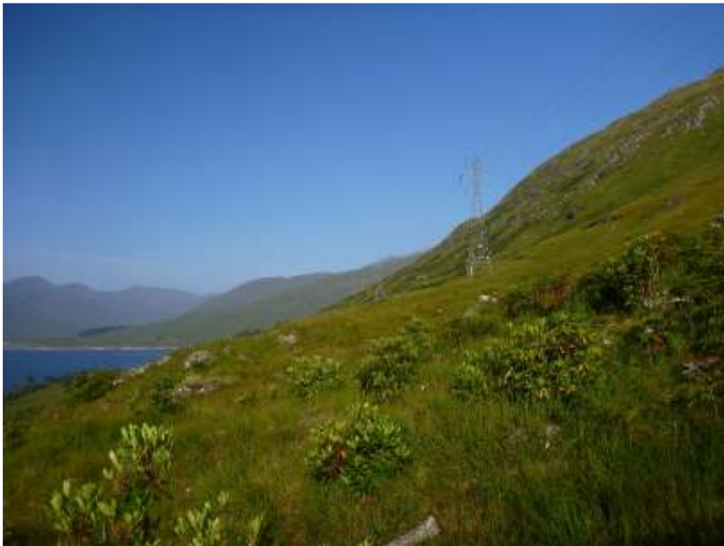
Skye transmission line looking west
