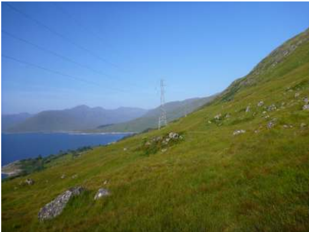
West along Skye transmission line
