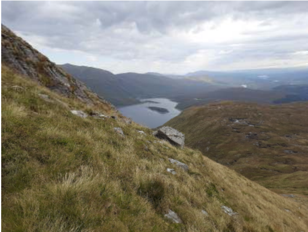
Looking towards Quoich dam, Fearna dam not visible
