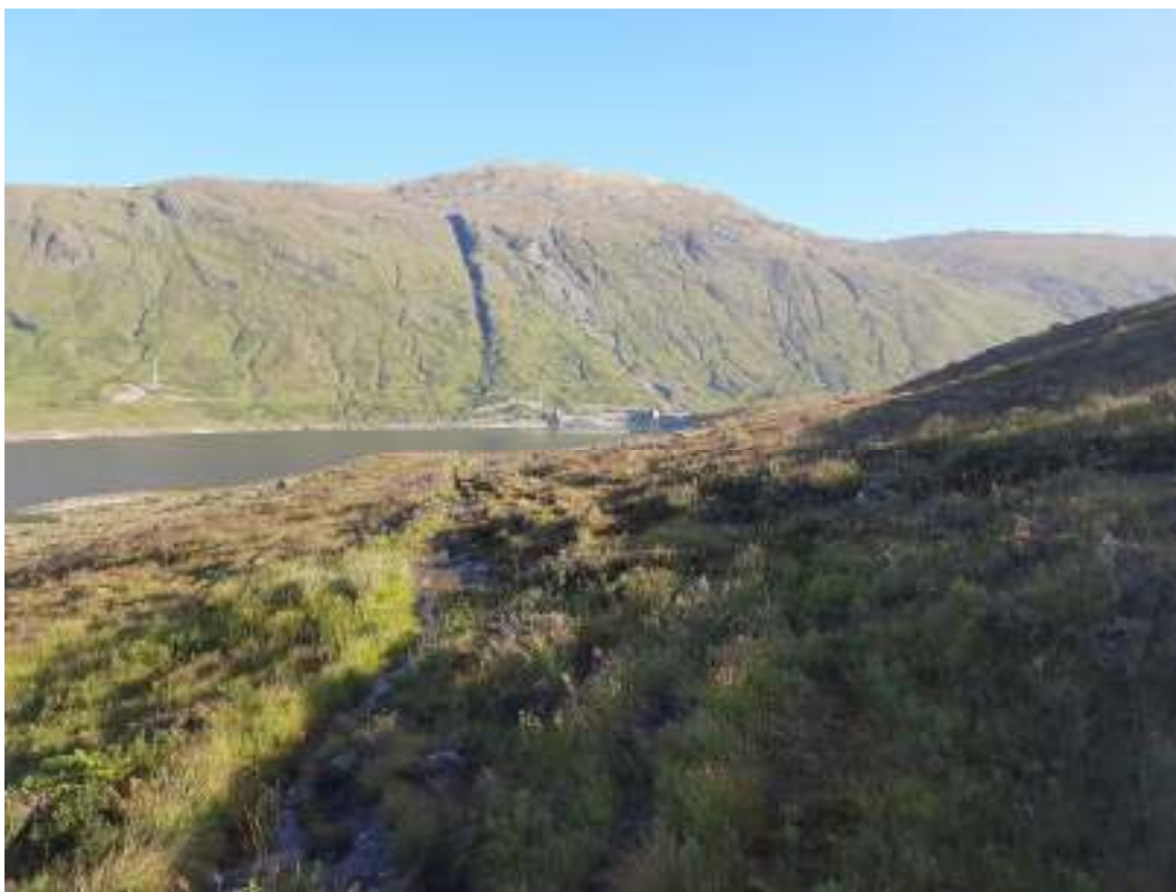
View towards Quoich dam
