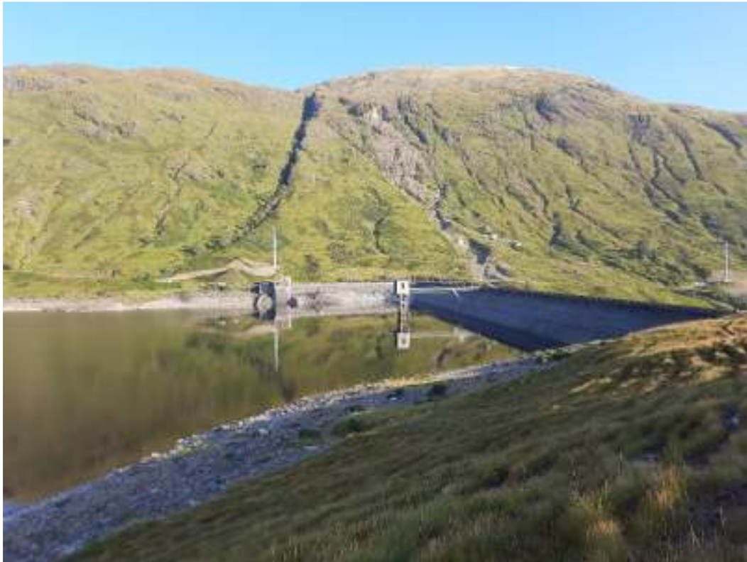
Towards Quoich dam and intakes
