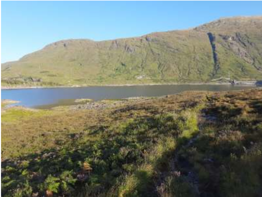
View towards Fearna Dam
