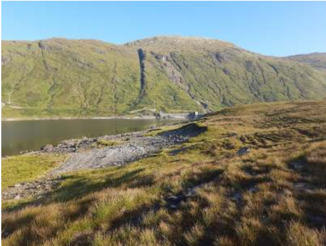
View towards Quoich dam
