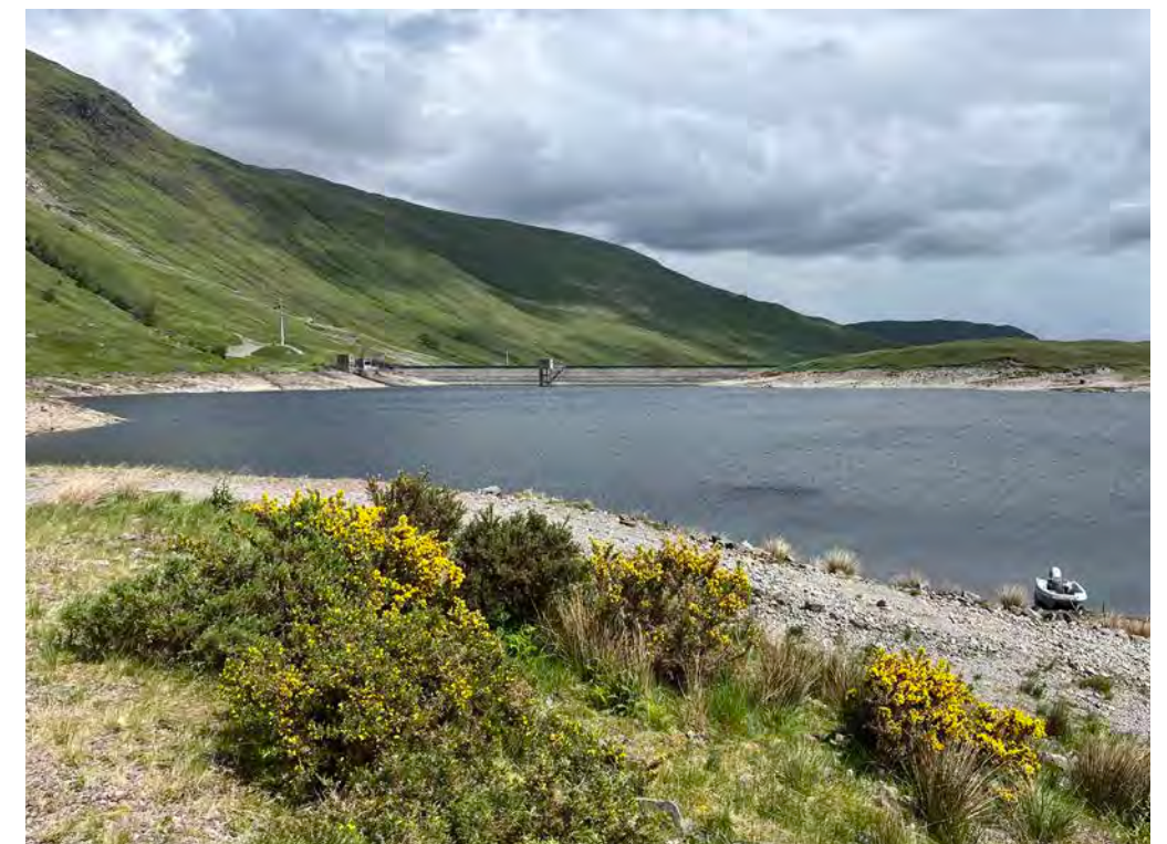
Figure 19 Existing Quoich Reservoir and HV transmission line from the proposed powerhouse site
