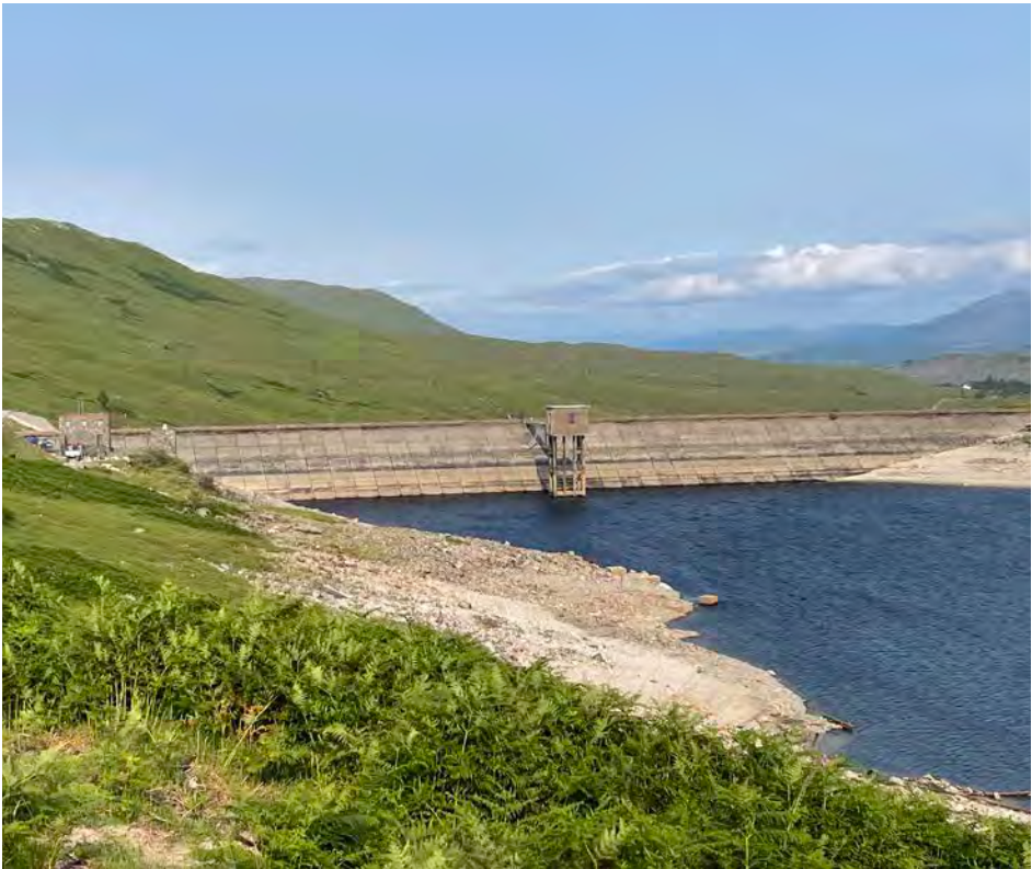
view looking eastwards to Quoich Dam
