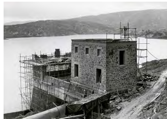
Figure 10 - North of Scotland Hydro-Electric Board Quoich Dam control building under construction (1956)
