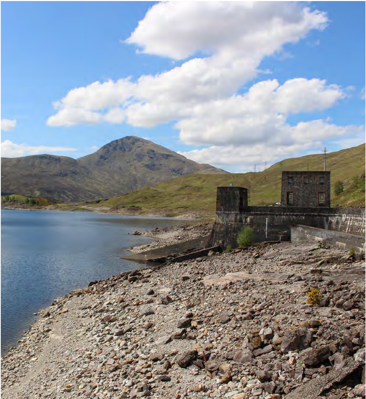
View from Quoich Dam westward towards Quoich control building
