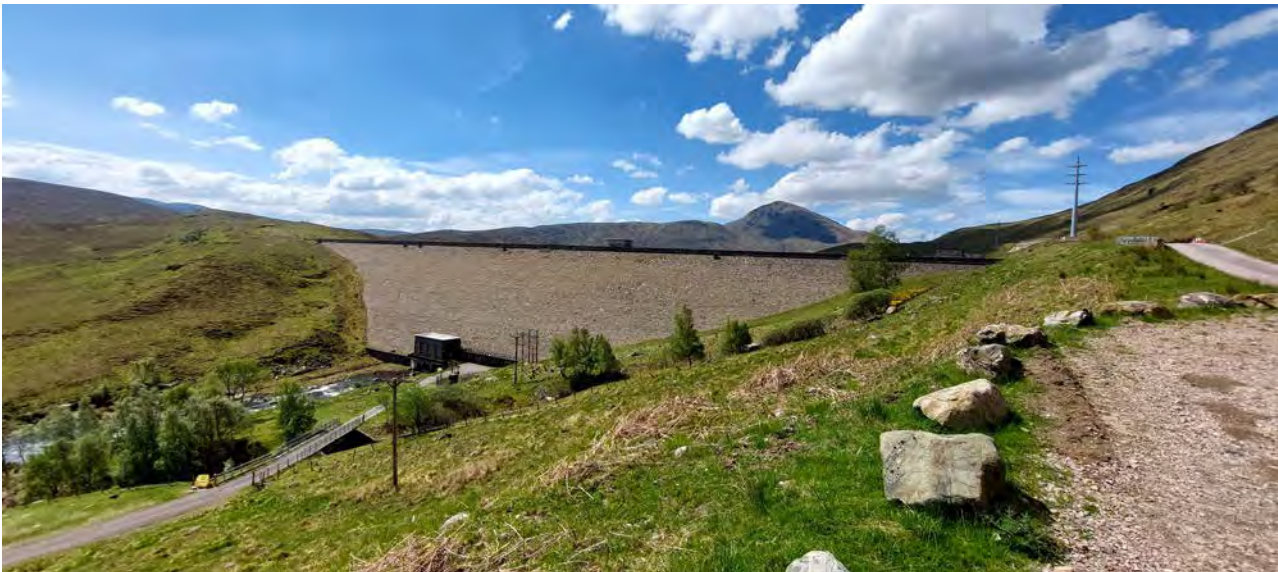
view of Quoich Dam and downstream valve house
