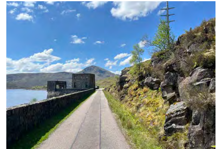
Figure 11 Quoich Dam control building, stone walls and existing rock face
