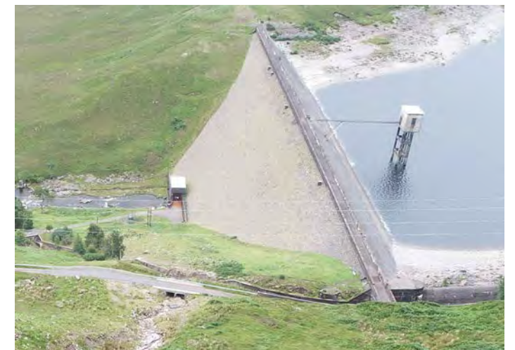
Figure 12 Quoich Dam - view from above
