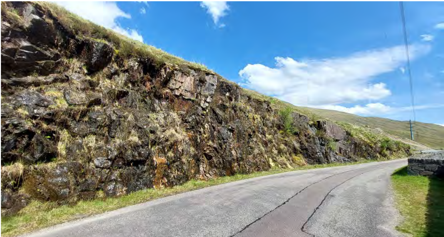
view of road cutting along the shoreline
