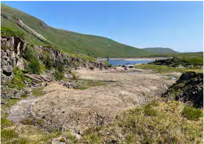
Figure 25 The disused quarry, looking east and partially infilled with 2018 landslide spoil (landslide visible in top left of image)
