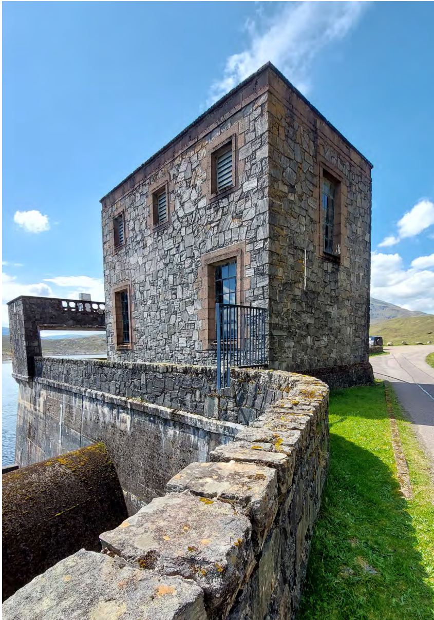
Quoich dam control building
