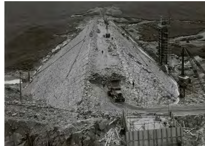
Figure 09 - North of Scotland Hydro-Electric Board Quoich Dam construction looking south (1955)
