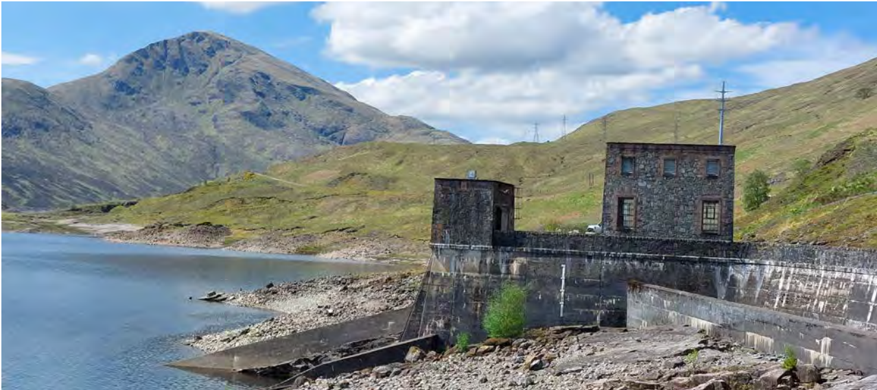
view of Quoich dam control building with proposed powerhouse site beyond
