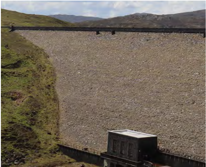
Loch Quoich Dam - east face
