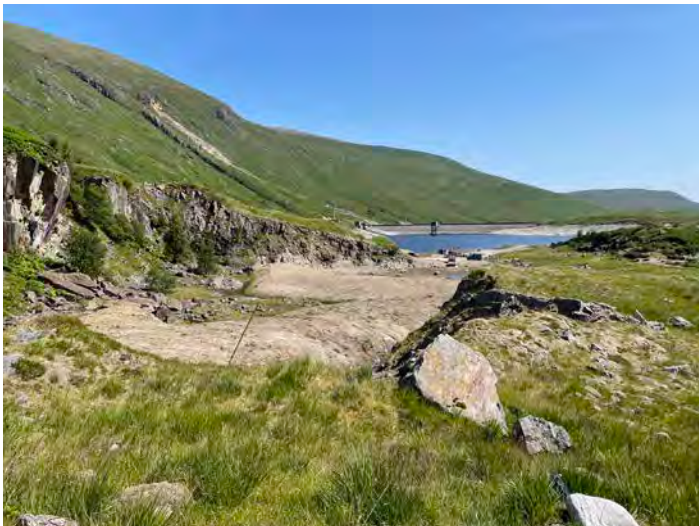
05 View towards Quoich Dam from disused quarry
