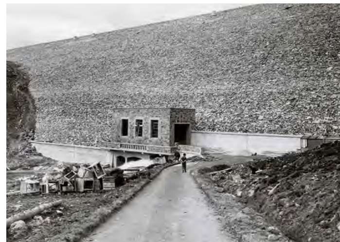
Figure 08 - North of Scotland Hydro-Electric Board Quoich Dam during construction (1956)
