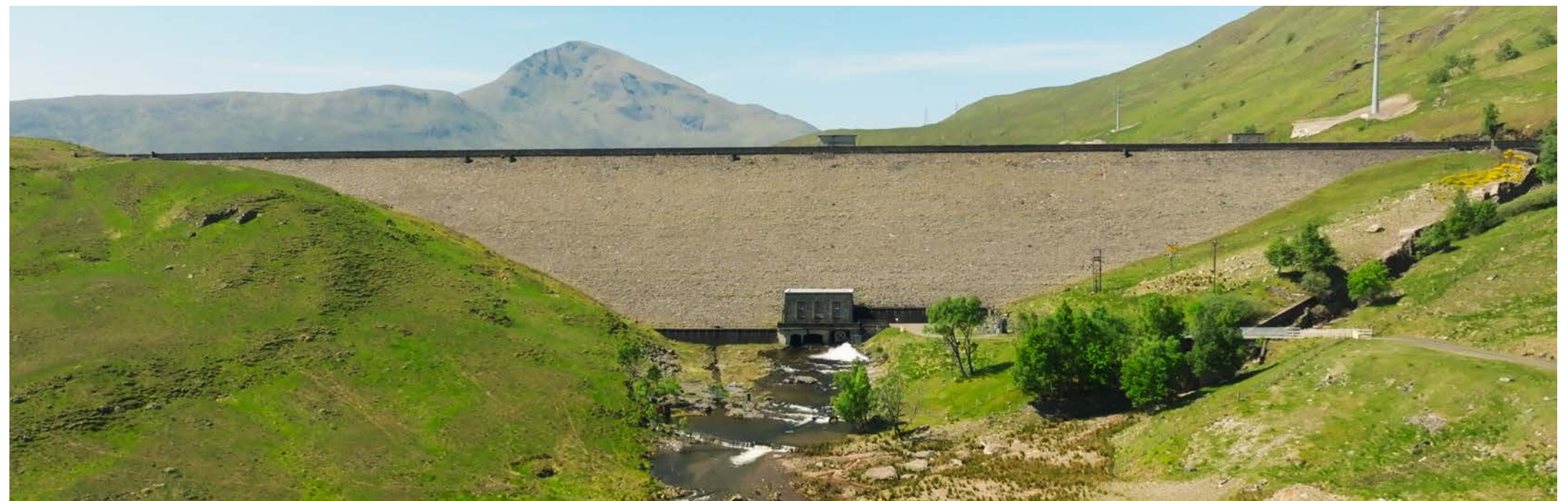
Figure 13 Quoich Dam - view from the east
