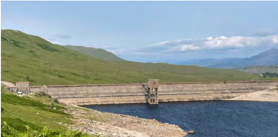
view looking eastwards to Quoich Dam
