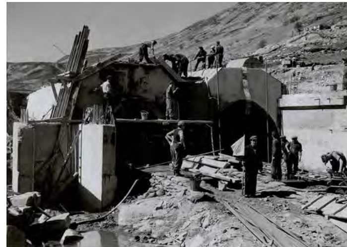
Figure 07 - North of Scotland Hydro-Electric Board Early stage of Quoich Dam construction - "The Hydro Boys" (1953)
