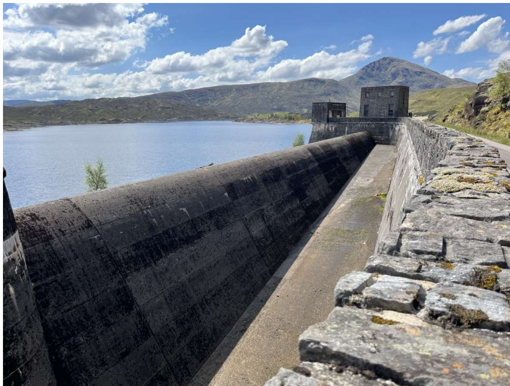
Plate 5 - Quoich Dam spillway and channel
