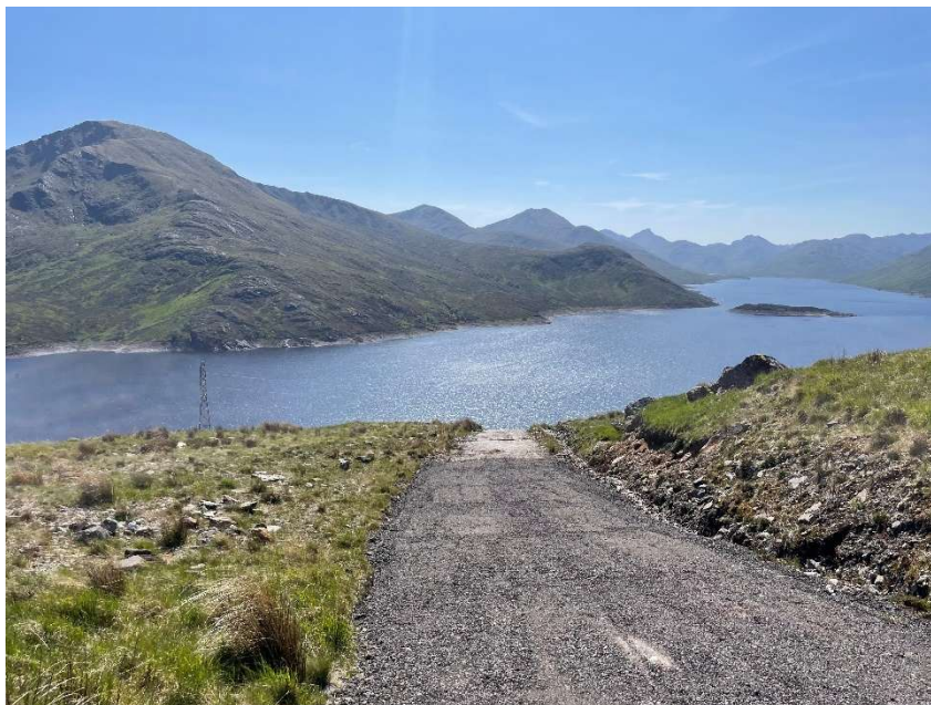
Plate 7 – Poor reinstatement, steep gradient and lacking drainage
