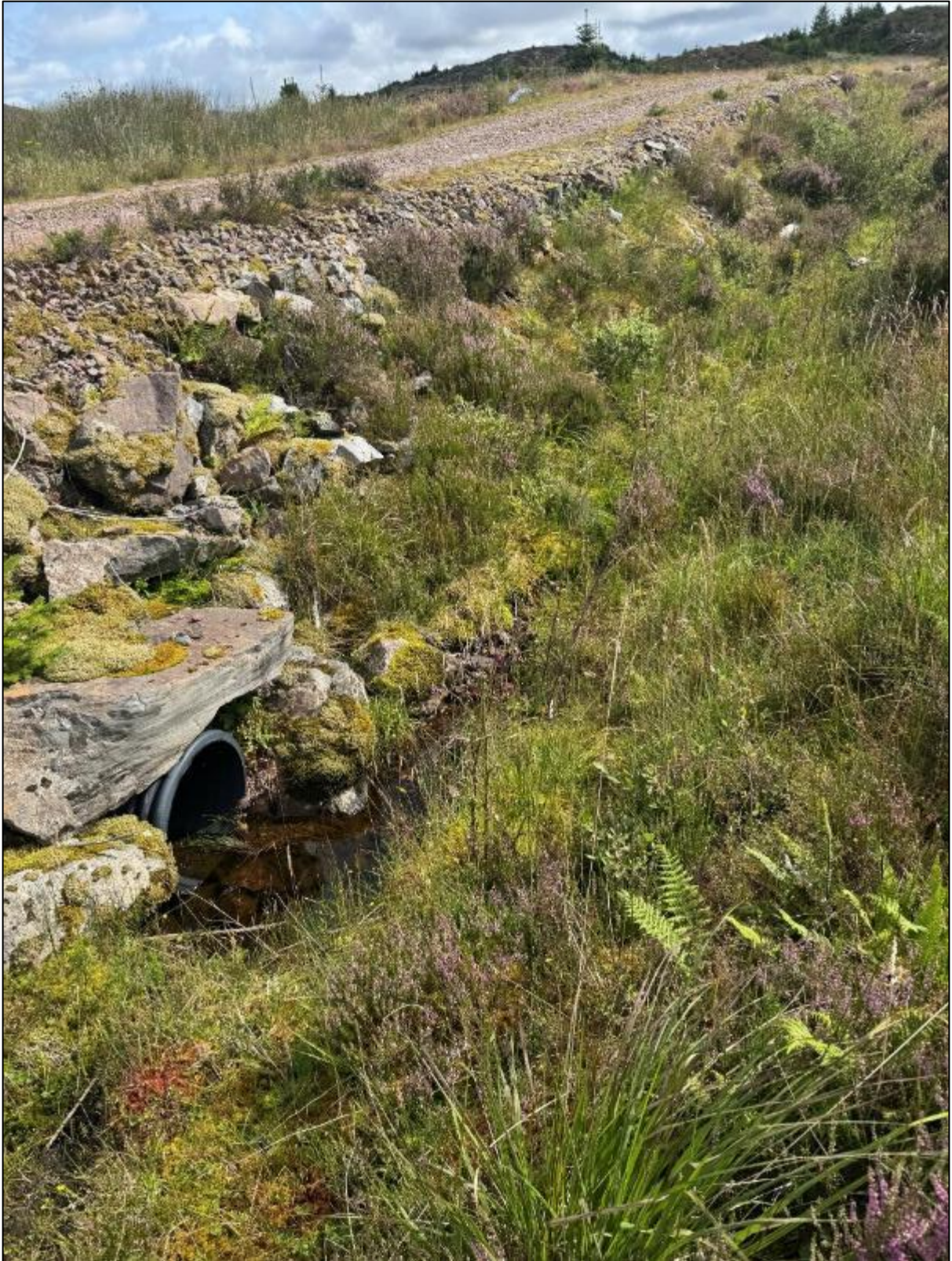
Figure A34. Photograph of stream crossing 34. Culvert entrance.
