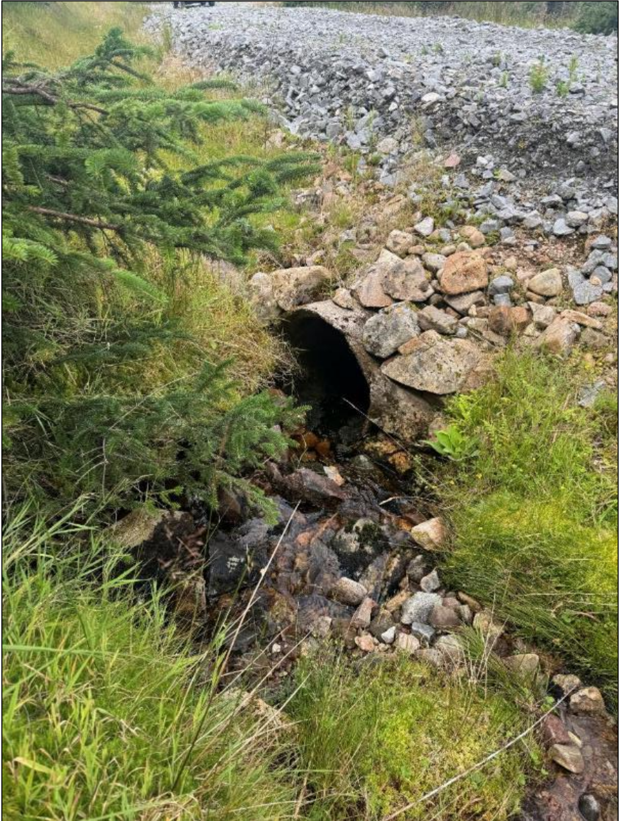
Figure A37. Photograph of stream crossing 37. Culvert entrance.
