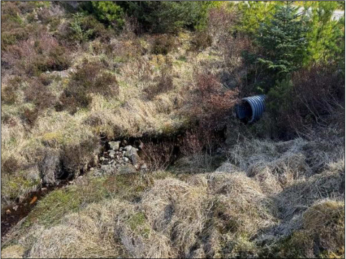
Figure A6. Photograph of stream crossing 6. Culvert outfall.
