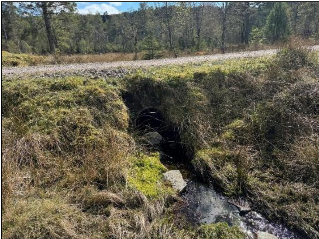
Figure A23. Photograph of stream crossing 23. Culvert outfall.
