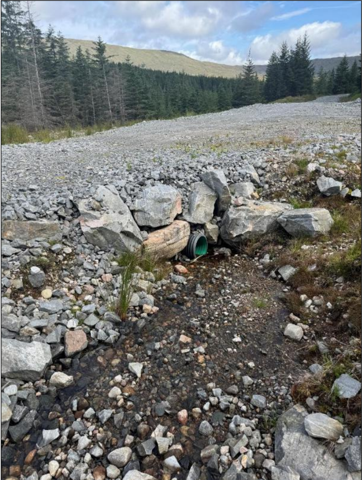
Figure A40. Photograph of stream crossing 40. Culvert entrance.
