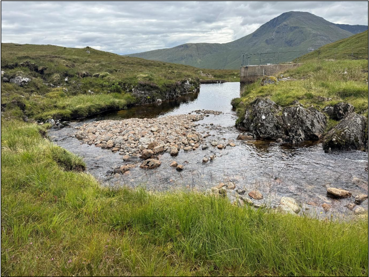
Figure 11. Alluvial sediment deposit located at the small hydropower intake structure on the Allt a Mheil at OS NGR NH 0465 0315.
